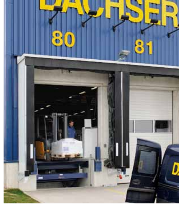
The lift leveller is a combination of a telescopic lip dock leveller and scissors lift table
